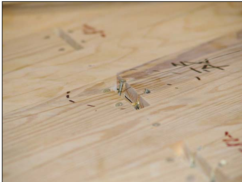
Figure 4.24 Butt-splice spreading, nail withdrawal and nail tear-out at sheathing board end (DDR = 1.5 %)
