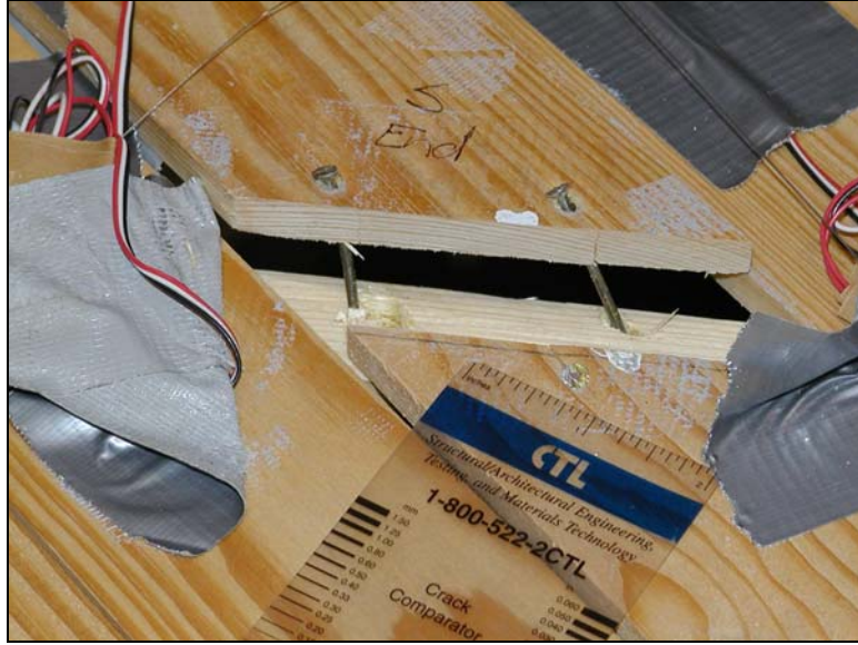
Figure 4.26 Nail withdrawal at maximum diaphragm drift ratio (DDR = 2.3 %)
