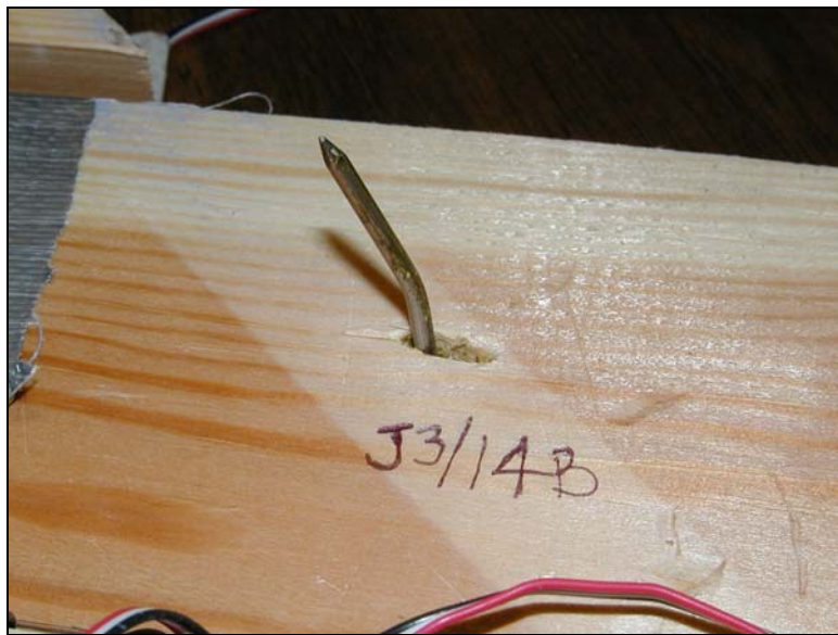
Figure 4.30 Typical deformation of nail and wood at nail hole
