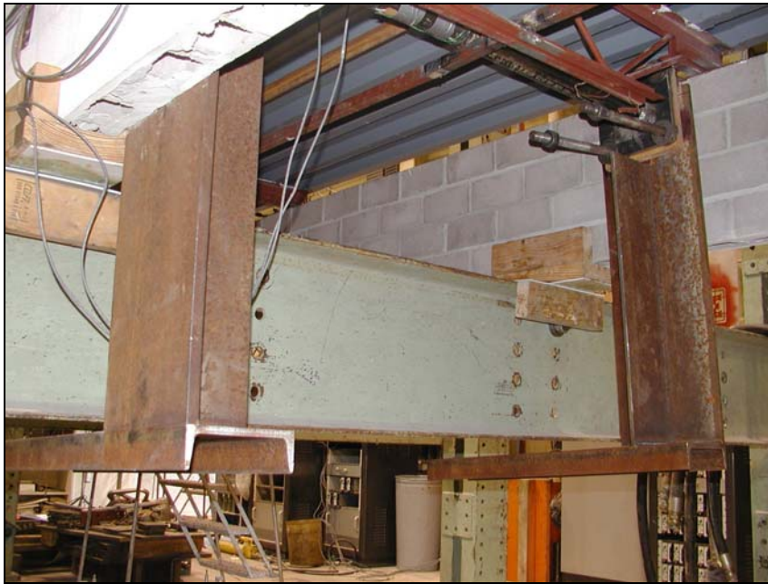
Figure 4.11 View beneath Diaphragm #2 at south channel showing L-shaped restraining members
