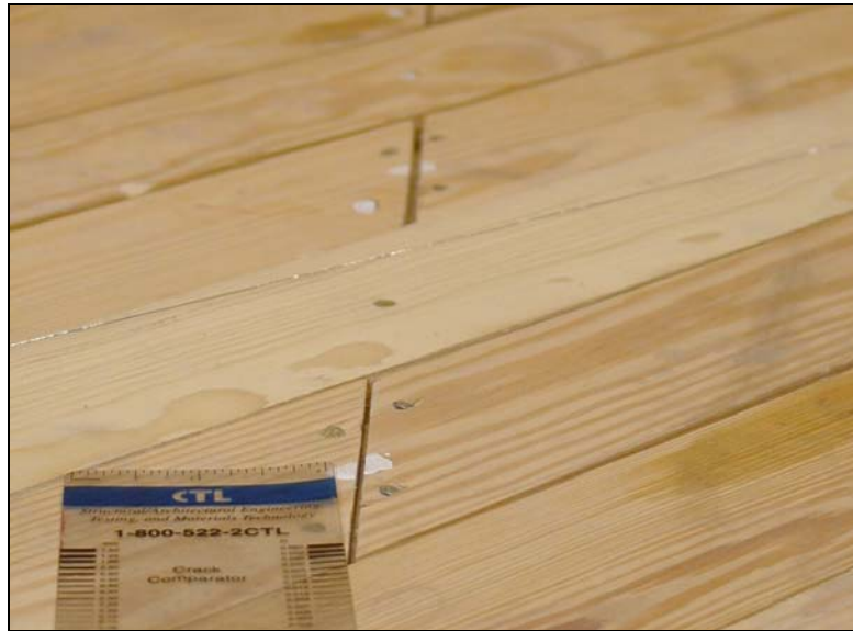
Figure 4.15 Spreading of butt splices under tension (DDR = 0.3 %)
