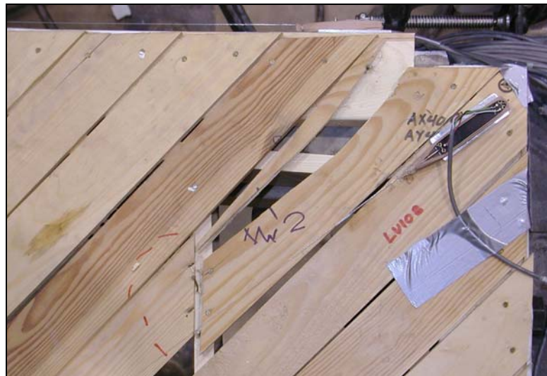
Figure 4.22 Severe damage to diaphragm, due to mechanism described in Figure 4.21 (DDR = 2.3 %, northwest corner)
