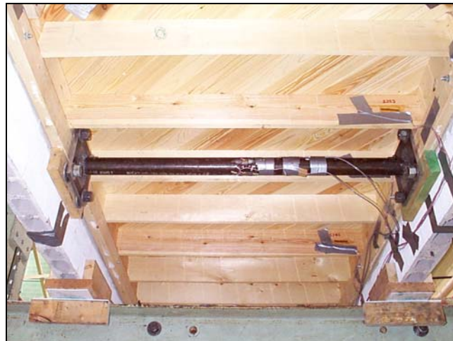
Figure 4.4 View beneath Diaphragm #1 showing load strut connecting east and west masonry chords at load points (similar for Diaphragm #2)
